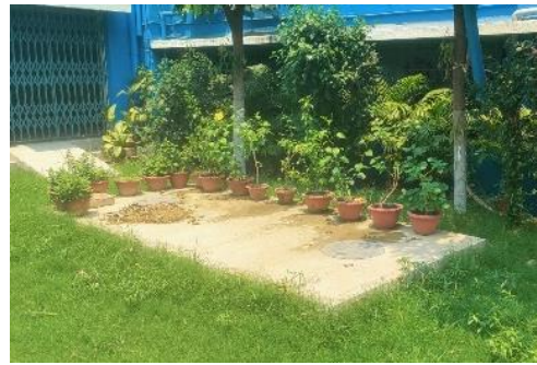
Chemical Waste Treatment Pit
